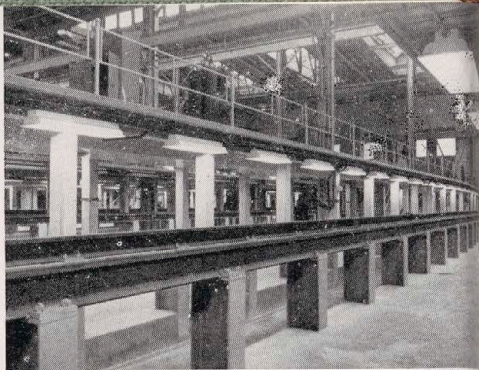
Five, 185-foot "pits" are provided for diesel locomotive overhaul work.
