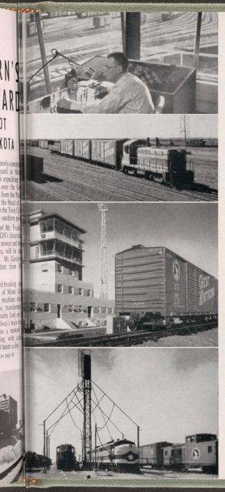
RETARDER OFFICE on the fourth floor of the control tower overlooks the yard and is the center of humping and classification operations. Controls enable the operator to manually modify any retarding maneuver he wishes.
