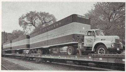
Part of a fleet of 40-foot vans and 85-foot flat cars of the Great Northern are shown being loaded in St. Paul for shipment of general commodities via piggyback. Two vans are accommodated on each flat car and are loaded in compliance with weight regulations in various states. They are part of GN's improvement program assuring fast, safe shipments along its more than 8,000 miles of track.
