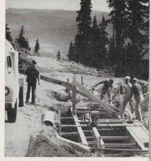
Concrete is shown being poured into forms of one of the landings of the new 6,800-foot double chairlift on the mountain. This site soon will be under feet of powder snow.
