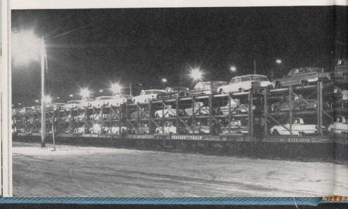
steel ramp facilitated loading of the top decks of the tri-levels. These decks carried station wagons which require slightly more clearance.
