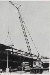
A derrick, provided by the Spancrete firm, easily sets the slabs in place. The firm also provides engineers to assist construction.
