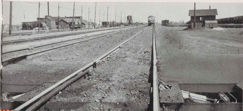
Two retracted journal box oilers are seen at trackside—each placed to service journals on both sides of the cars.
