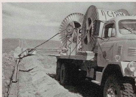
Handled gingerly by an experienced machine operator, above, the reels of cable soon find their way to the "back country" below, where they are laid into a missile site network
