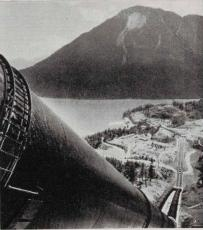
Bridge river water is carried by mile-long penstocks, above, to Hydro's bridge river No. 2 powerhouse. Cleveland dam, left, on the Capilano river provides much of the water to the Vancouver area.
