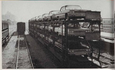
A fully-loaded Trailer Train tri-level is shown at the car facilities at Renton, Wash. The equipment carries 15 standard-sized automobiles.
