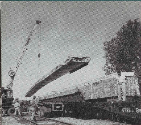
A crane operator gingerly lifts a giant beam off the gondola and prepares to ease it onto a waiting truck bed.
