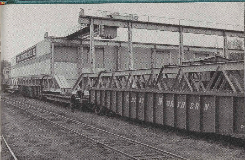
More than 133 tons of steel trusses, fabricated by the St. Paul Structural Steel Company of St. Paul, left there recently on Great Northern Railway flat cars bound for the College of Great Falls at Great Falls, Mont. The huge trusses, 12 in all, will be used in the construction of a recreational center. Six are 115 in length and the others 86 feet. They were loaded three abreast for shipment.
