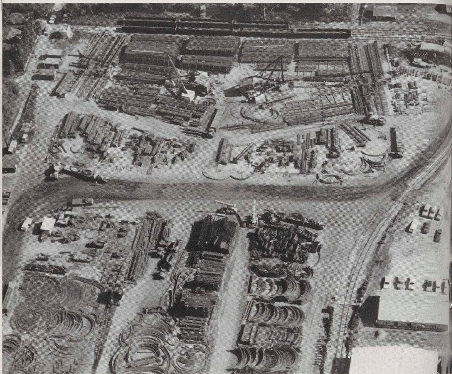
Massive piles of various shapes of steel bars, plates and sheeting are visible in this aerial photo of the American Bridge Division's yard of U.S. Steel at Grand Forks. They are components of silos which house Minuteman Missiles.
