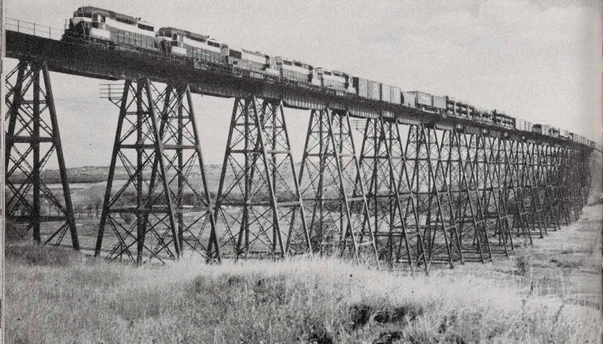
The striking profile of a modern freight train—powered by five giant diesels—is seen on a high trestle on GN's main line west of Minot, N.D. The trestle, spanning Gassman Coulee, is 117 feet high and 1,792 feet long.
