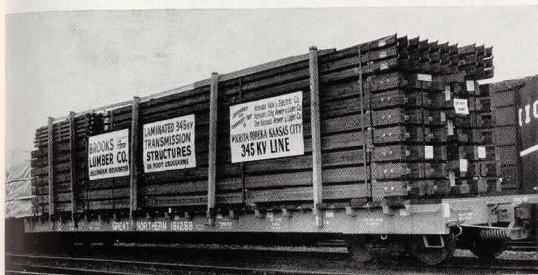
Brooks Lumber Company of Bellingham, Wash., recently shipped 56-foot laminated cross arms for 345 K.V. power line to the Kansas Power & Light Co. of Bazar, Kansas. The shipment moved on GN to Laurel for connections to Kansas. Also involved in the flatcar movement were the Kansas City Gas & Electric Co. and the Kansas City Power & Light Co. Gross weight of the freight was 133,500 pounds.
