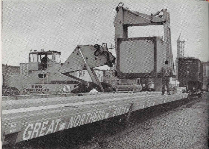
In Seattle, "Piggy Packer" loads a 20-foot sealed container on one of GN's new TOFC/COFC flat cars.
