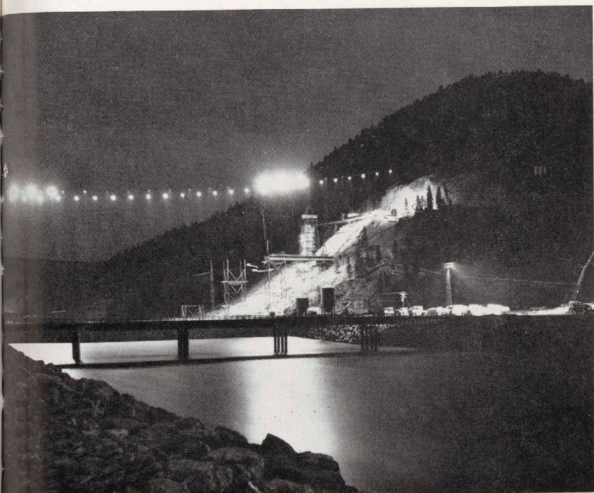
Libby Dam construction area at night. Work trestle is a major construction job in itself.
