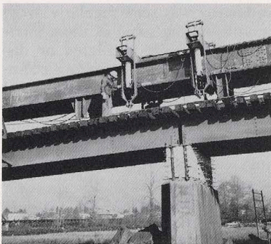
Four slabs have been placed on this pier. Raise is about half completed at this point.
