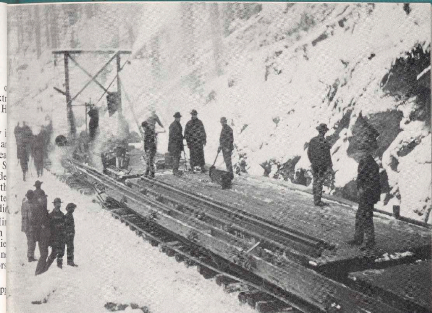
December 10, 1892. Using a unique track-laying machine, workmen are laying the last segment of main line west of the Cascade Range summit.
