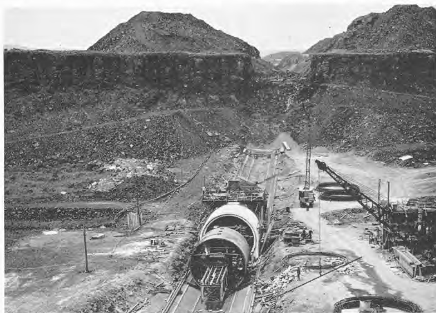
Building the 1,000-foot Bacon siphon, on the main canal of the Columbia Basin Irrigation project. Can you find the man in the foreground? The siphon is over four times as high as he is. It will carry water across a natural depression and will connect with Bacon tunnel, a 10,000-foot bore through lava rock. Siphon and tunnel together, are costing $3,494,000. In the background, the main canal, from the north, is shown in rimrock.
