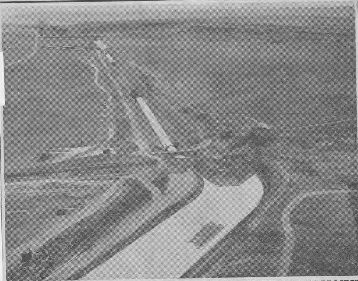
AERIAL VIEW SHOWS WEST CANAL AND SIPHONS ON COLUMBIA BASIN PROJECT
