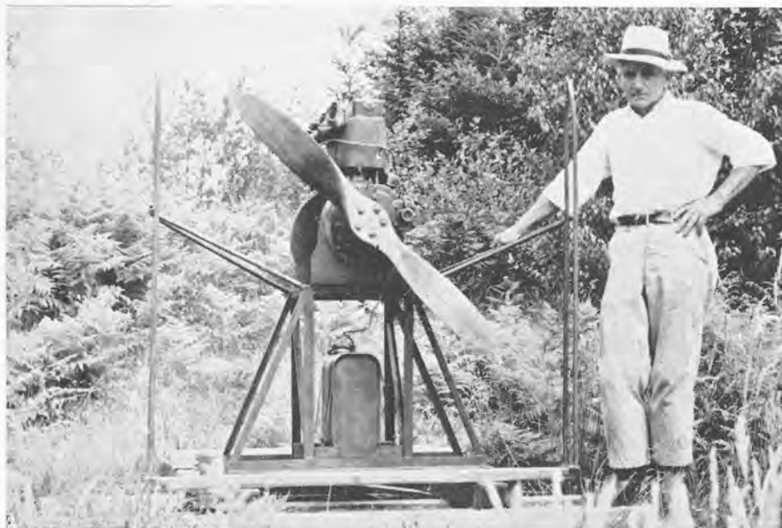
Joseph Eberhardt, in Thurston county, Washington, has three large propeller-type fans, like this one, placed at one end of his planting of tame blueberries and along one side, on ground that is higher than the peat soil his fruit occupies. Sometimes it gets frosty in the bog when it is 12 degrees warmer on nearby higher ground. A thermostat in the middle of his blueberry field sets off a bell at the house when the temperature hits 34 degrees. After this warning, Eberhardt turns on the fans, which push out cold air and suck in warmth from the higher land. In three years he has had the fans, frost damage has been avoided. His story is told on page 3.
