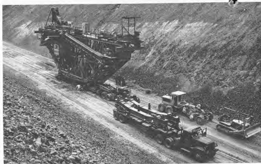
This kind of equipment is used to trim and line, with concrete, open sections of the large canals on the Columbia Basin Irrigation project. Six and a half miles of the west canal have been lined with concrete. Bids are to be requested soon for lining some six miles of the main canal and the first 12 miles of the east canal, which eventually will be 130 miles long, are being lined now.
