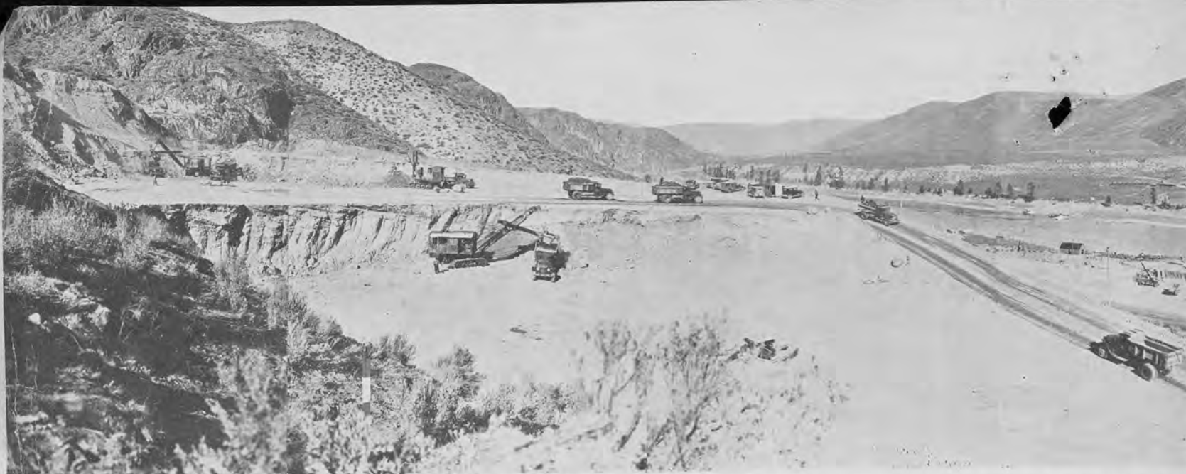
Here is the first panoramic view of operations at Coulee Dam. This picture was taken by Pacific Builder and Engineer February 23, 1934, when the David H. Ryan contract for preliminary removal of overburden was about 50% completed. On the near side of the river is Schedule No. 1, subject to Goodfellow Brothers Inc., Wenatchee. Average haul from excavating area (left) to spoil bank (right) is 2500 feet. On far side of river is Schedule No. 2, M. S. Ross and Rowland Construction Co., subcontractors. Average haul to spoil bank at right is about 2,200 feet. Note test trench just above the excavated area. It marks the axis of the dam.
