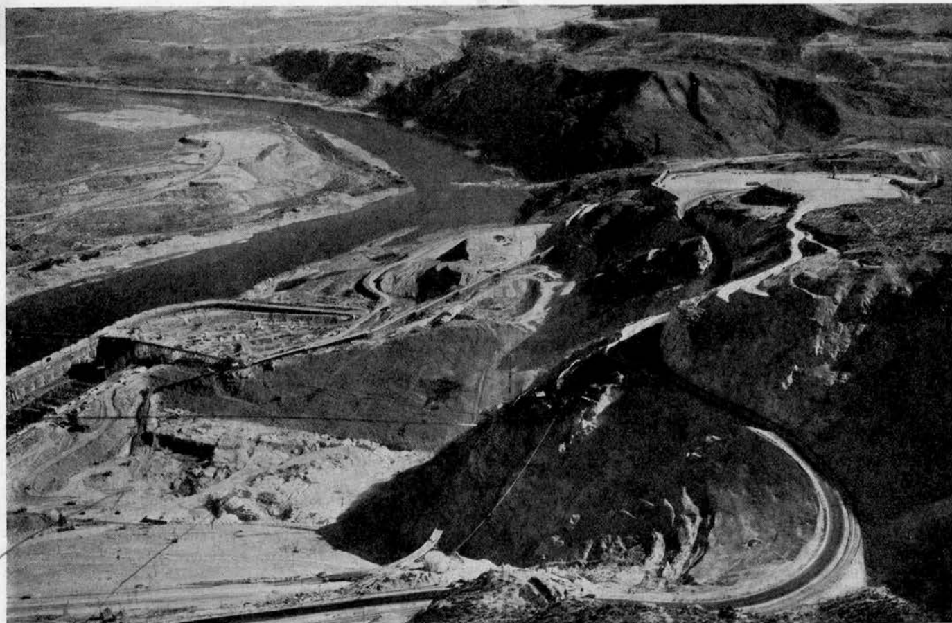
The new Government highway circling down into the gorge of the Columbia at the Grand Coulee Dam site. In the background, along the Columbia, is shown a part of the huge curving cofferdam behind which excavation is almost complete for the foundations for the west abutment of the dam.
