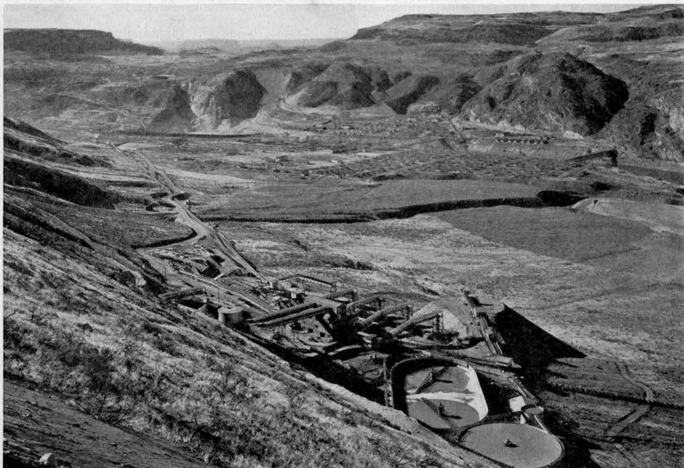
The huge clarifiers and the gravel crushing and screening plant downstream from Mason City and the Grand Coulee Dam site. The second big conveyor of the Mason-Walsh-Atkinson-Kier Co. carries the aggregate from this plant to cement mixing plants, one on each side of the Columbia, down into the vicinity of the huge cofferdam which can be seen faintly, encircling the white excavation area in the background of the picture. Mason City, the contractors' all-electric town, is shown in about the center of the picture, and across the river is the Government engineer's town. The Columbia, flowing as it does between steep banks, is hidden in this view, although it divides the two cities.
