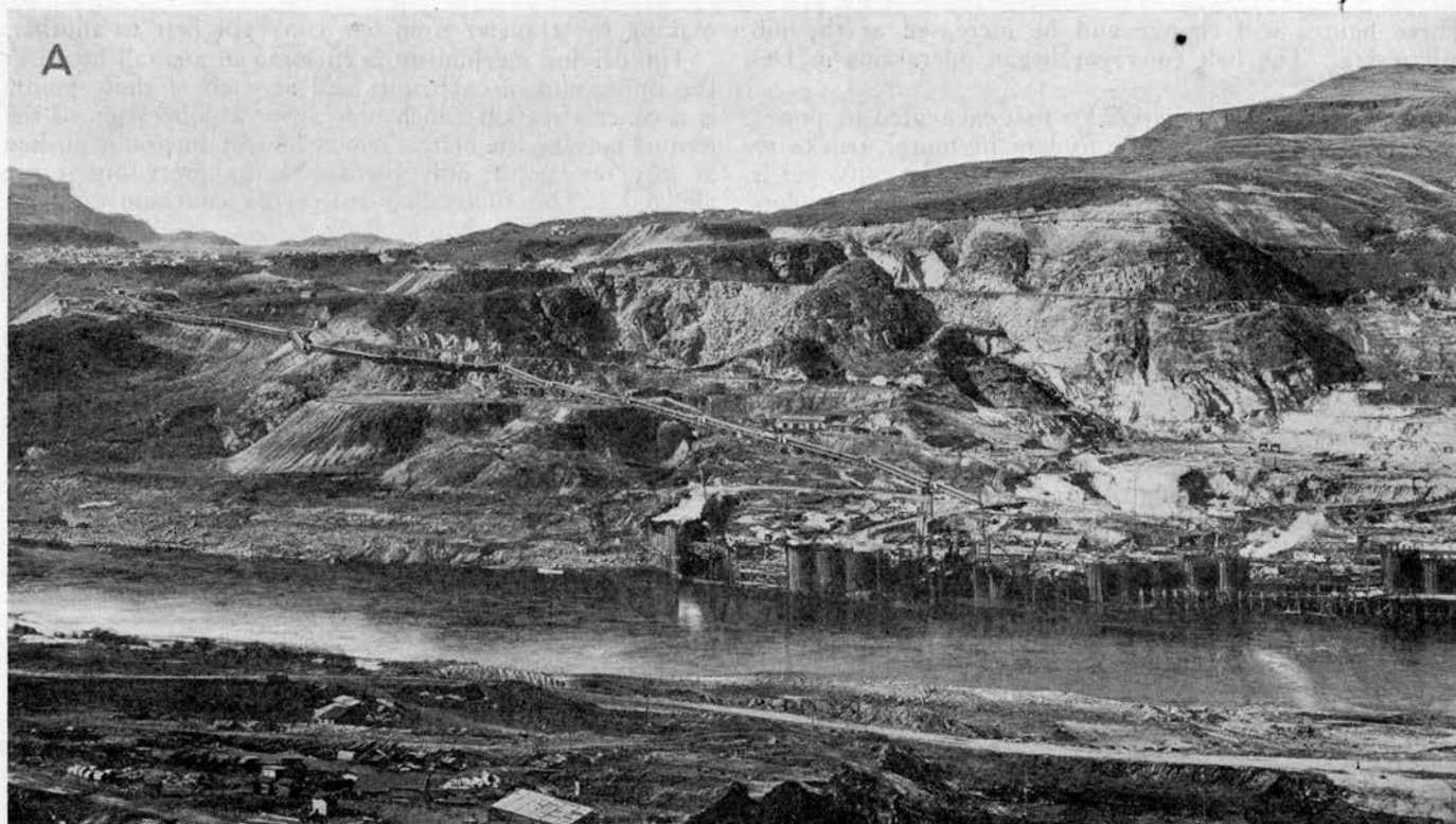
A view of the cofferdam at the Grand Coulee when still under construction. Climbing the hill behind is the snake-like structure of the big conveyor and high on the cliffs are some of the mushroom towns, reminiscent of the old West, that have grown in the wake of the huge construction project.
