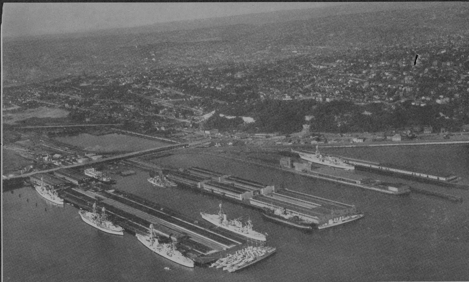
PIERS 40 and 41, the great terminals of the Seattle Port Commission. These are the largest piers of this type in the world. All piling used in the construction of these piers is Creosoted Douglas Fir.
