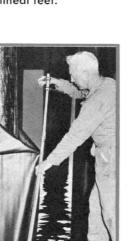
PILE-GARD encircling pile, ratchet in position ready for wrapping operation.
