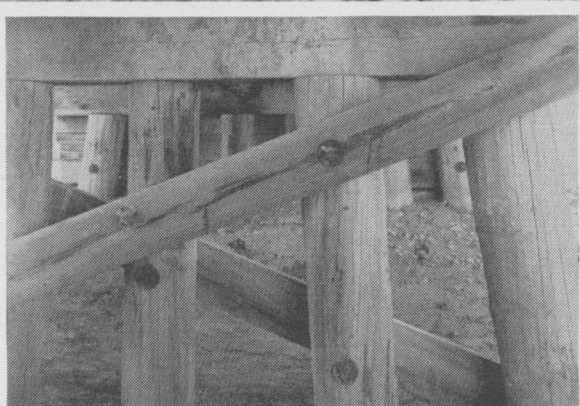
THIS CLOSE-UP of part of Bent 3, Bridge 259-A shows original piling, sway brace ends, cap and flooring.
