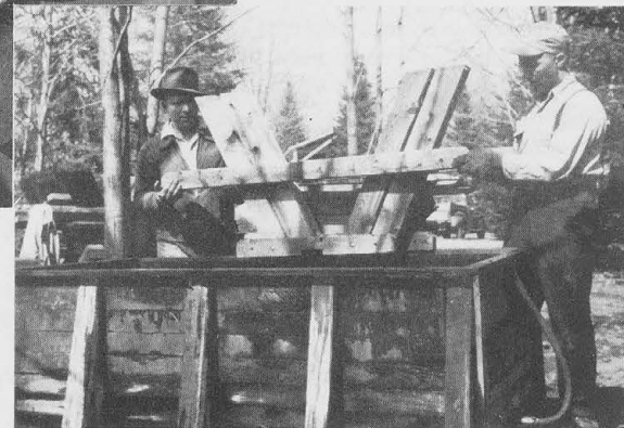
After the bench legs are assembled they are treated in a water-repellent solution containing "penta."
