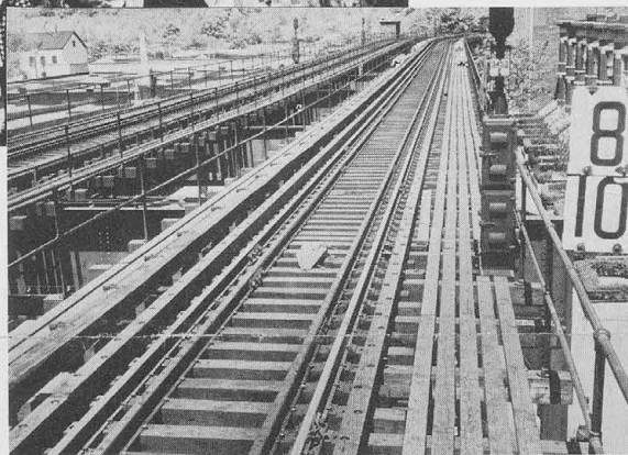
Looking up Track No. 2 on the New Lots Avenue BMT elevated line in Brooklyn. Clean "penta"-treated crossties are used over street crossings and on open viaduct structures to protect traffic from possible drippage below.
