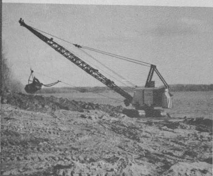
Dike construction and repair are the history of Lake Chautauqua
