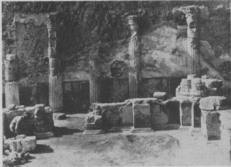
Section of lower terrace, Herod's northern palace—plaster-on-stone columns, wall paintings simulating stone and marble.
