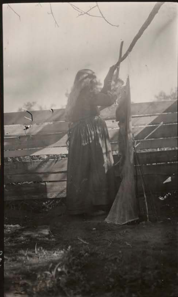
(b) Placing deer hide in position over frame
