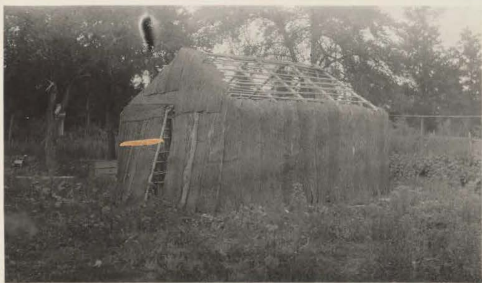
III. 76 Partially completed structure to be used for mat weaving
