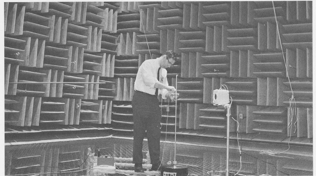
H. S. Knoll sets up equipment as it might be used for a test inside the Acoustic Facility's anechoic room, where thousands of glass wool wedges absorb sound.
