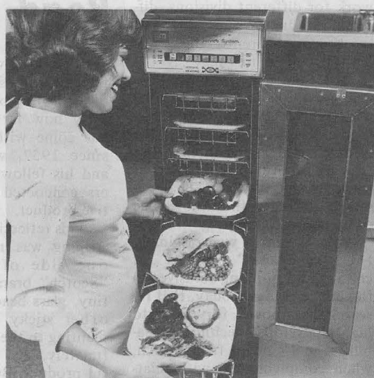
ELECTRONIC "memory unit" in the "Integral Heating" control module allows different kinds of foods to be heated at the same time, each receiving just the amount of heat it needs.
