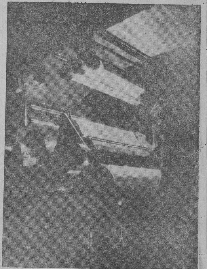
INSPECTION — Richard Scheff watches carefully as the jumbo rolls of sasheen ribbon wind up as they come out of the dyeing and aligning machine. The 36-inch wide roll is inspected here for flaws or imperfections. These large 36-inch rolls are the final product of the company's maker department.
