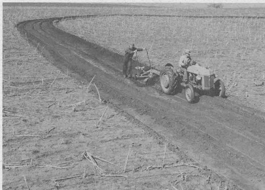
Constructing channel-type terrace with 6-foot Texas terracer and Fordson tractor in Oklahoma
