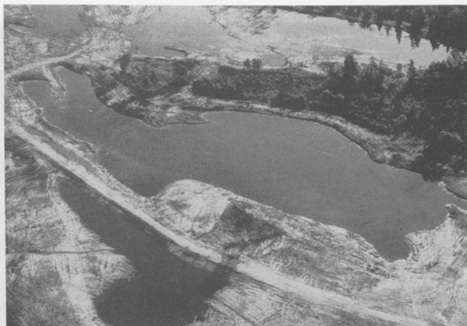
Fig. 4. Excavation of borrow from the Lake George Borrow Pit resulted in a series of basins that will eventually become a wetland complex.
