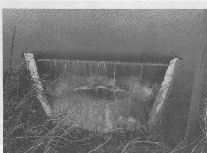
Fig. 2. Spring runoff flows over the culvert outletting Lamperts Marsh. Before the elbow was added, much of this water drained off, leaving the marsh in a seasonally wet condition.
