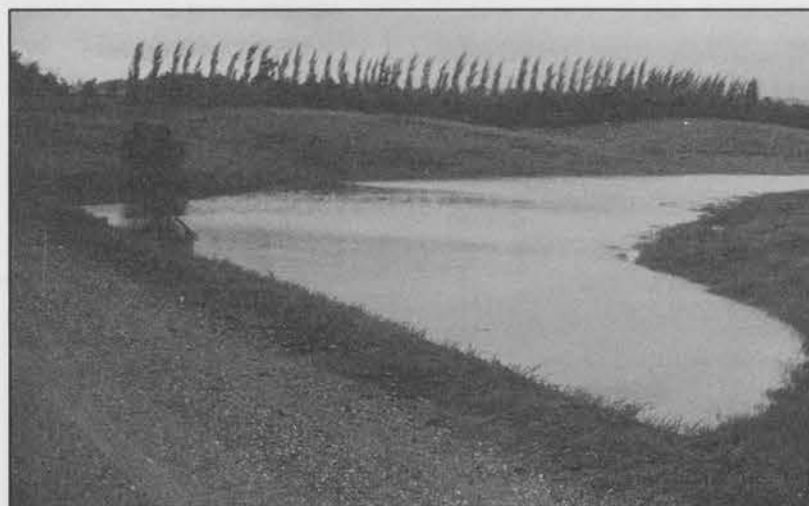
Road retention projects use roads to provide temporary upstream floodwater storage to reduce downstream flooding.
