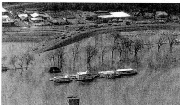
BWSR's St. Paul office is located off to the photo's left edge.
