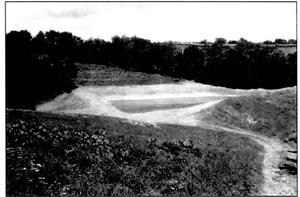
4. Grade Stabilization Structure
