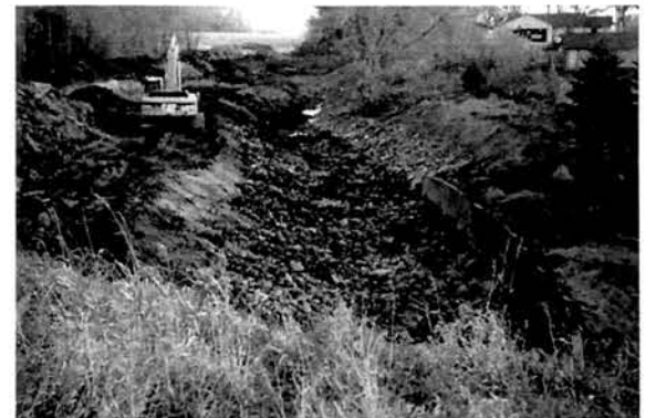
Ditch repair was made to correct erosion problem on CD-32 in 1999 (after).
