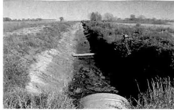
CD-37 after the ditch was cleaned out (2000).
