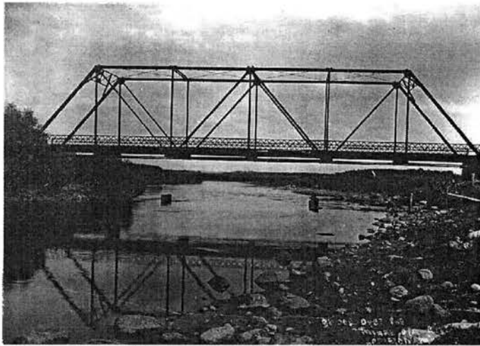
Swift County Bridge over the Minnesota River, 1905
