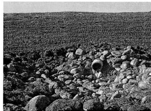
SW Sportsmens Club Small Dam Repair Lincoln County
