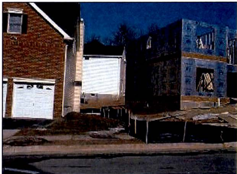
Permitted construction sites must identify and implement best management practices like the silt fences and ground covering seen here.
