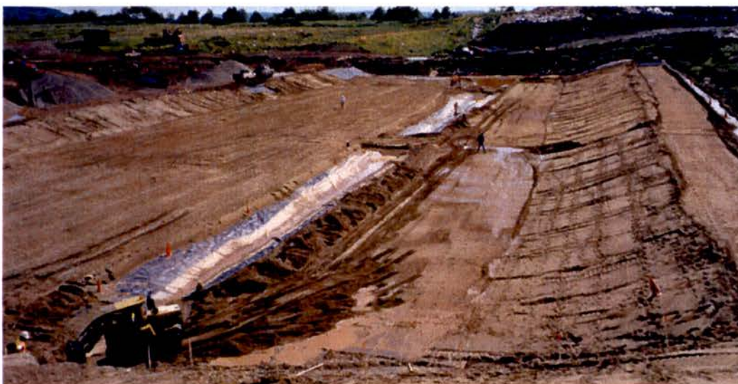
This photo shows the construction of a lined MSW landfill in St. Louis County. The liner is visible as a dark strip in the center. A layer of sand has already been applied over the remainder of the liner. The sand and liner keep liquid wastes from contaminating ground water.
