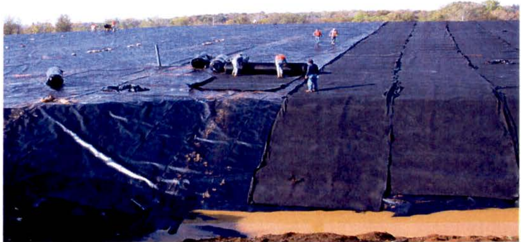
A synthetic liner is placed over waste at a landfill to keep rain and melting snow out. When water filters through the waste it becomes contaminated and will then contaminate surrounding land and ground water.
