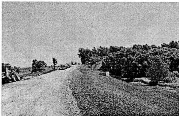
Normania 32 Bank Stabilization Yellow Medicine County
