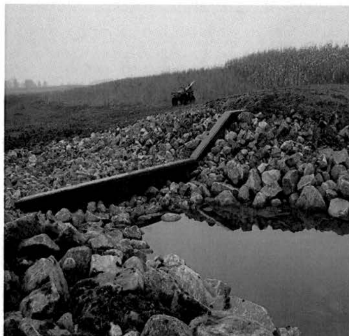
Constructed steel sheet pile weir outlet with plunge pool (wetland basin off to the left)
