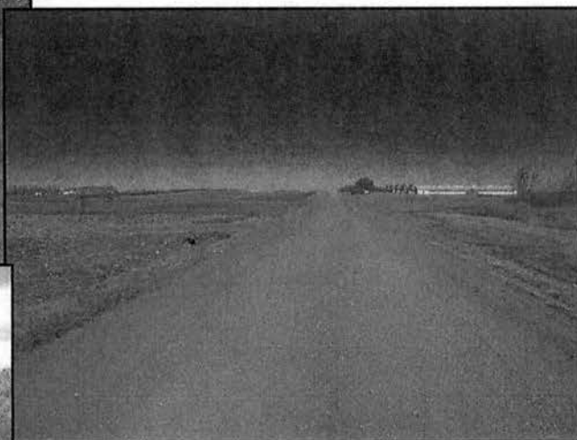
AMIRET 32/33 ROAD RETENTION (Lyon County)
