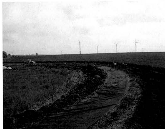
Construction of Denitrifying Bioreactor
