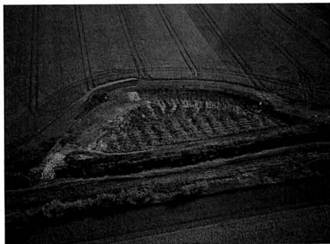
Aerial View of Detention and Treatment Basin
