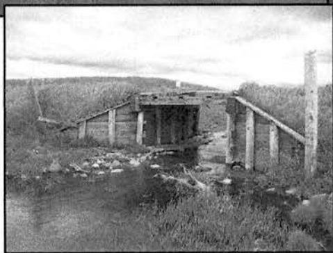
Replaced deficient bridge
