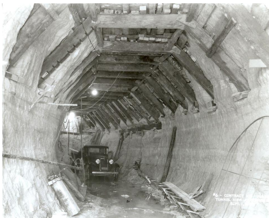
The furthest downstream tunnel constructed in the St Peter Sandstone exited St Paul's Dayton's Bluff north of Warner Rd east of its intersection with Childs Rd, which allowed entry of the vehicle. The Joint Interceptor section here is a 13'-10" circular sewer completed in 1935. About 1200' upstream from the location of this photo the sewer invert is 212' below the surface.
