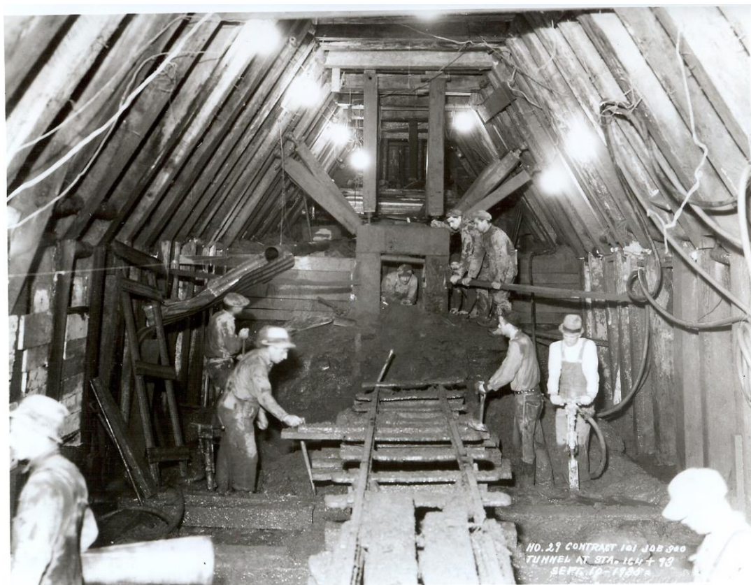
Seven workers are shown in the tunnel being constructed in the stream sediments of Glacial River Warren terrace east of downtown St Paul. At this location, about 112' below Lafayette Rd and Grove St, a 13'-3" semi-elliptical section of the Joint Interceptor sewer was constructed in 1935.
