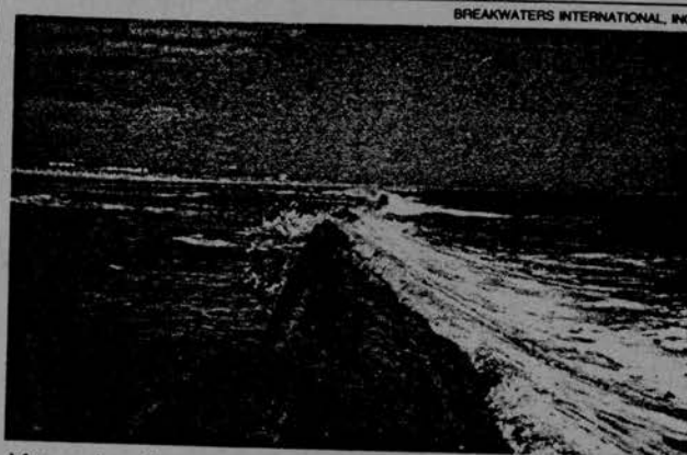
Man-made reef prevents erosion of beach; marine dwellers on the reef may be preventing pollution.
