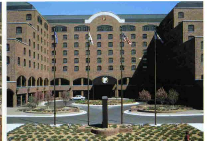
The Radisson University Hotel complements University of Minnesota campus and University Hospital activities.
