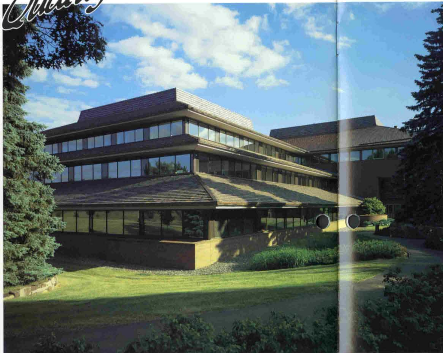
Projects for Cargill, Inc., include construction of its Minnetonka, Minn., office center—a 400,000-square-foot building and 164,000-square-foot addition, along with parking ramps for 1,700 cars.
