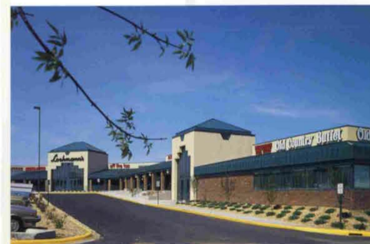
Loehmann's Plaza is a 209,000-square-foot shopping center in Roseville, Minn.
