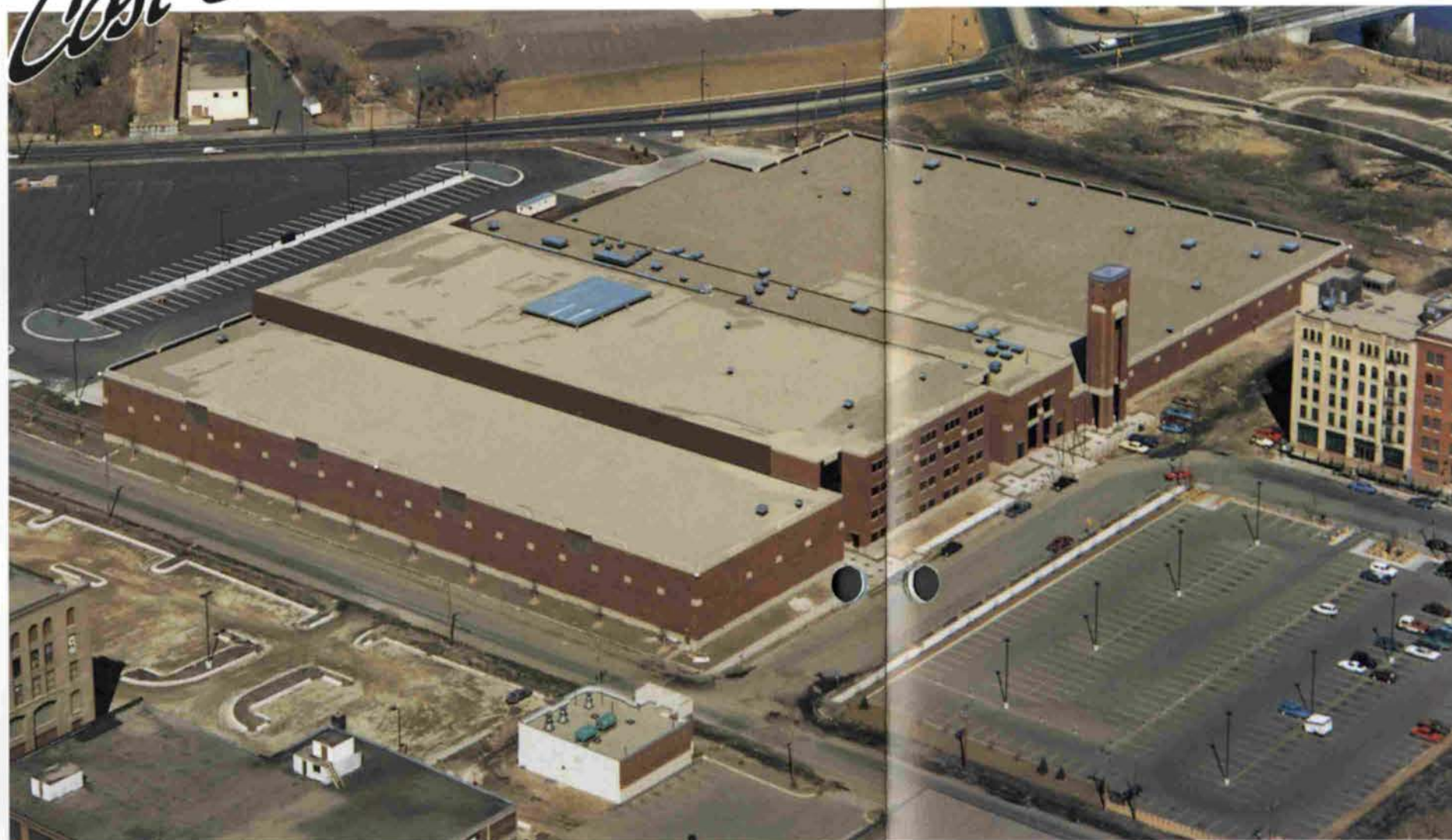
A 395,000-square-foot printing plant was built for the Minneapolis Star and Tribune near the Mississippi River in Minneapolis.
