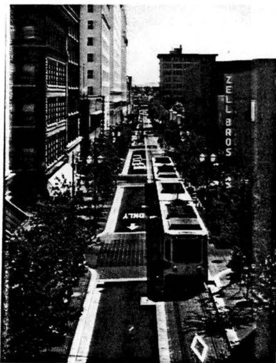
Special paving treatments can successfully delineate LRT, pedestrian and vehicular circulation areas, as demonstrated in Portland, Oregon.
