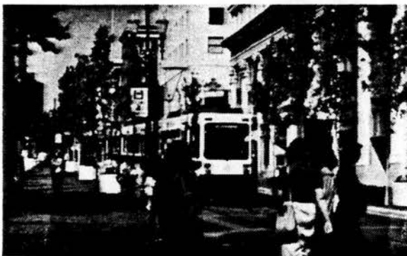
As in Portland, Oregon, trolley wires can be supported from ornamental light poles and buildings to minimize their visual presence.
