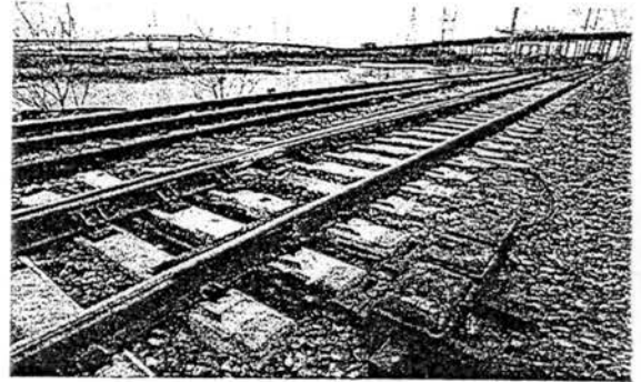
State-of-the-art track construction.
