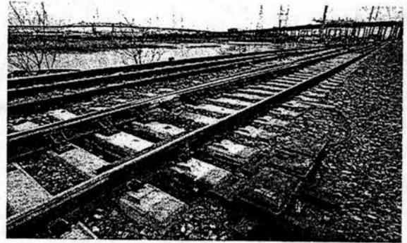
State-of-the-art track construction.
