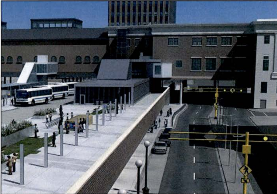
View of multilevel glass/steel structure from above the train deck.
