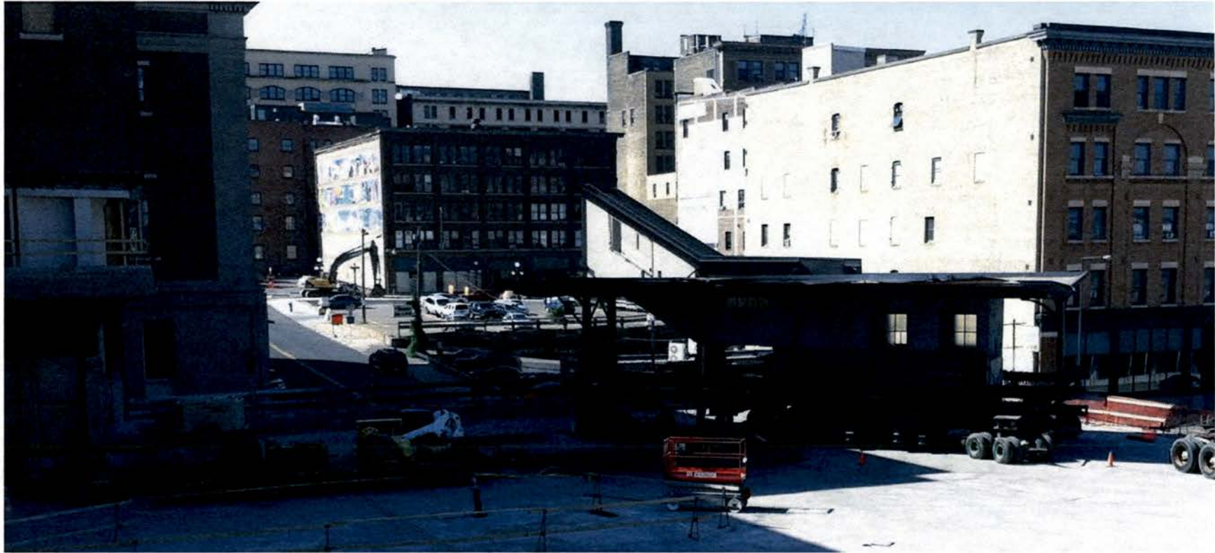
Historic Platform/Stair Relocation
