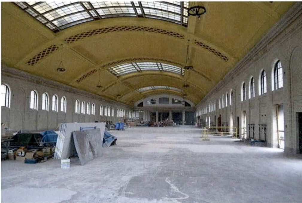
MAIN FLOOR: View of Waiting Room, looking north ( Under Renovation ) Dated: June 15, 2012
