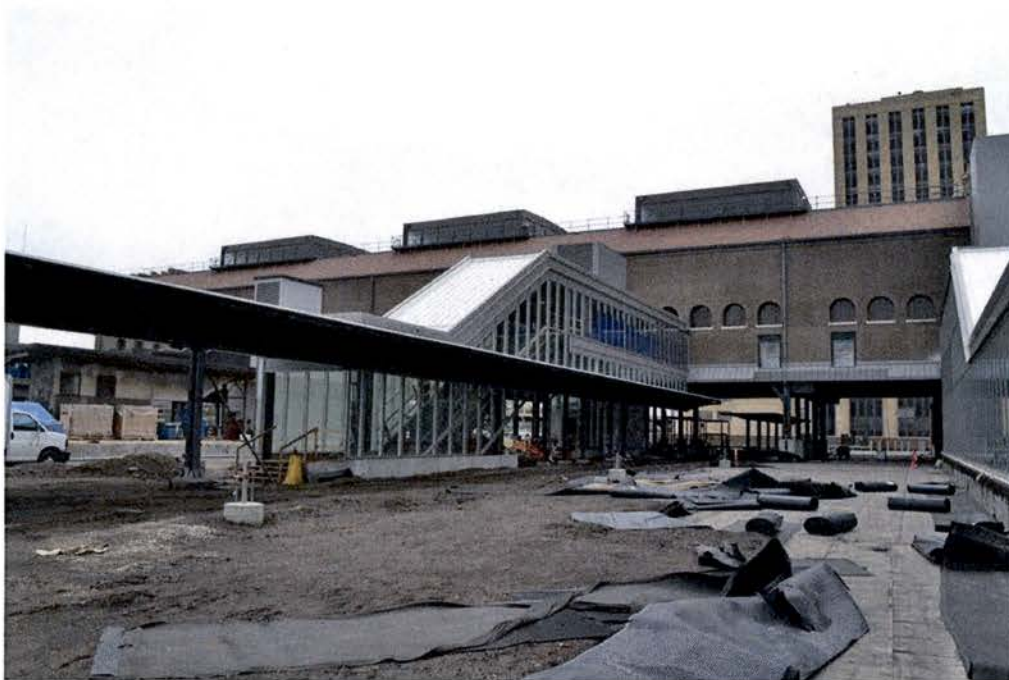
VERTICAL CIRCULATION TOWERS: Skyway Entrance in Head House Dated: June 15, 2012
