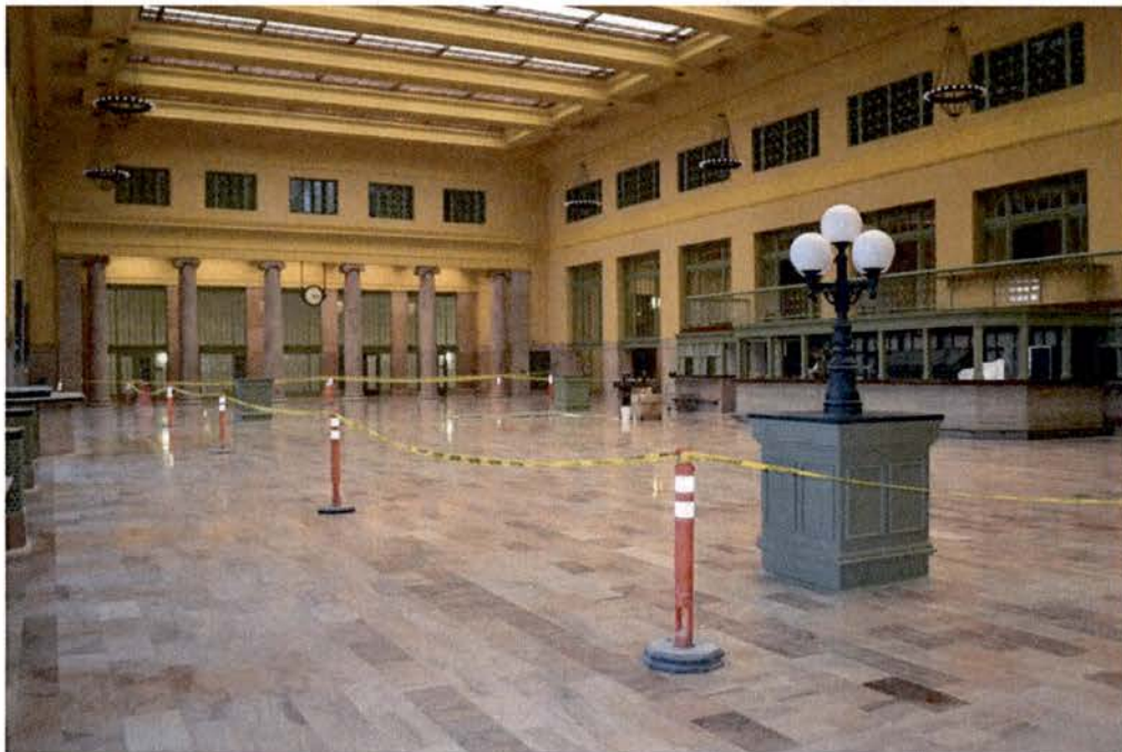
MAIN FLOOR: Tenant #1 located in Head House – Christos (Under Renovation) Dated: November 23, 2011
