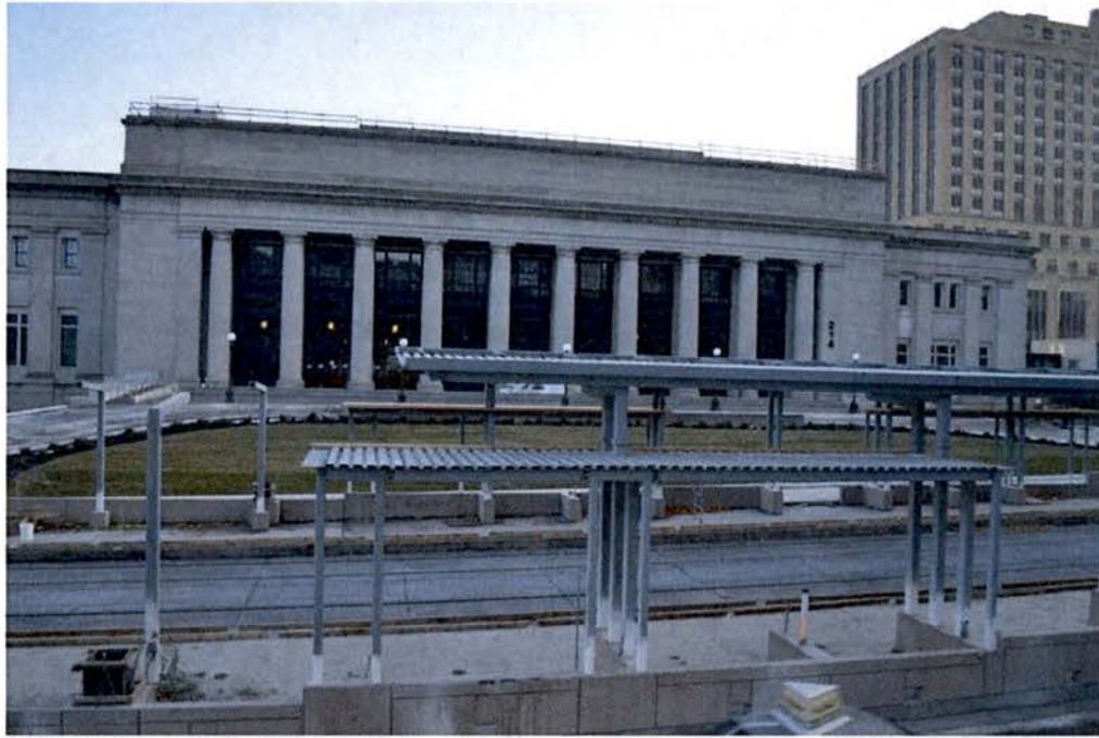
FRONT PLAZA: Light Rail Platform (Under Construction) Dated: November 23, 2011
