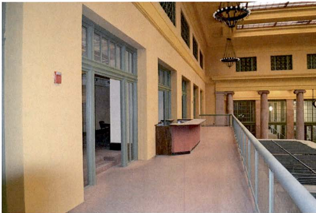
MEZZANINE: Tenant #11 located in Head House (Under Renovation) Dated: November 9, 2011
