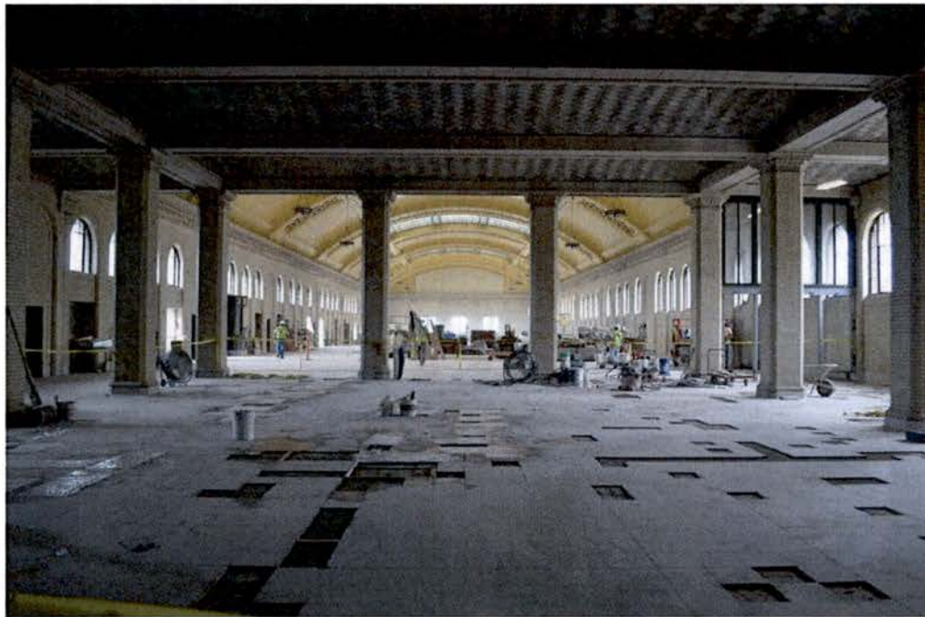
MAIN FLOOR: View looking south from Concourse (Under Renovation) Dated: June 15, 2012
