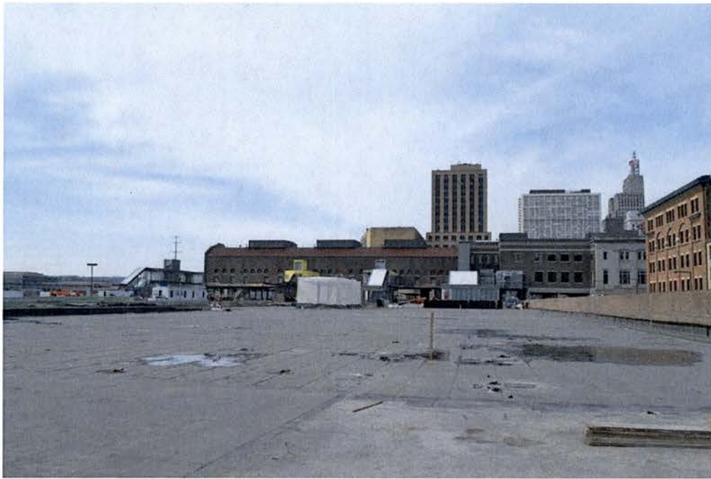
TRAIN DECK: Looking west towards Waiting Room Dated: (under renovation) March 6, 2012
