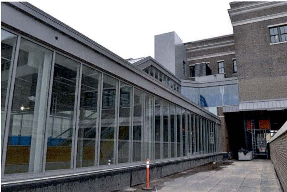
KELLOGG ENTRANCE: View of entry at train deck level ( under renovation ) Dated: June 15, 2012
