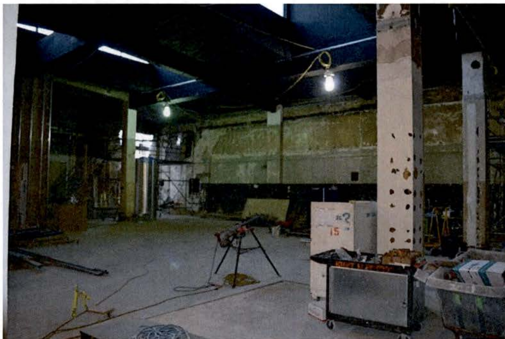
SECOND FLOOR: Tenant #9 located in Concourse (Under Renovation) Dated: November 9, 2011
