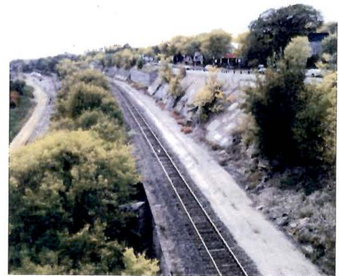
CP Rail mainline looking south from Smith Avenue
