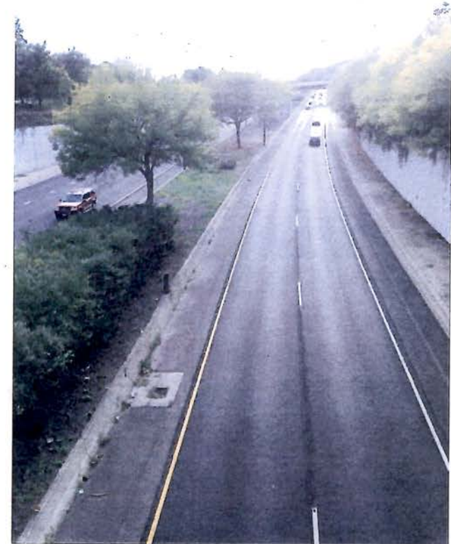
I-35E looking south from Grand Avenue
