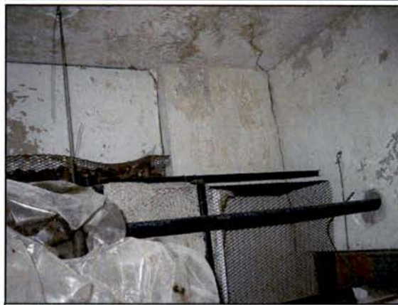
Mezzanine – Ceiling Plaster (Sample 3F)
