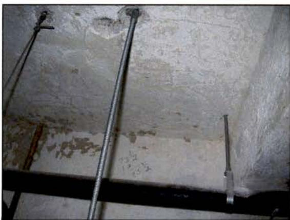
Mezzanine – Ceiling Plaster (Sample 3E)
