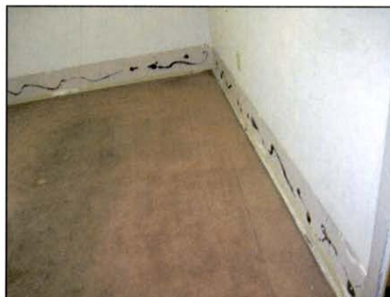
Mezzanine – Gypsum Board with Tape and Joint Compound and Black Baseboard Adhesive (Samples 8A and 20A)
