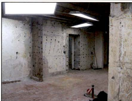
Column Plaster (Sample 3B)
