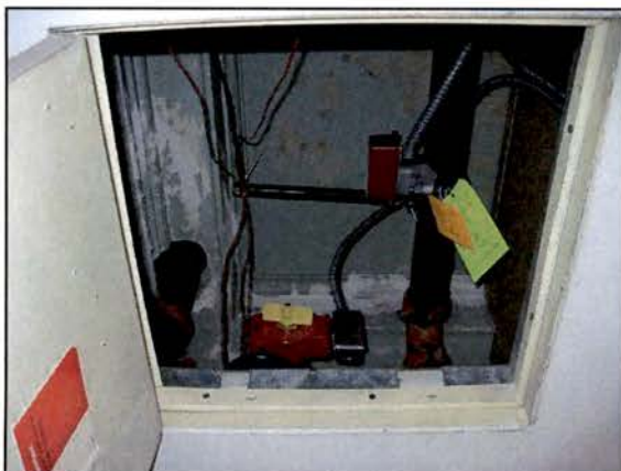
Mezzanine – Ceiling Plaster (Sample 3G)
