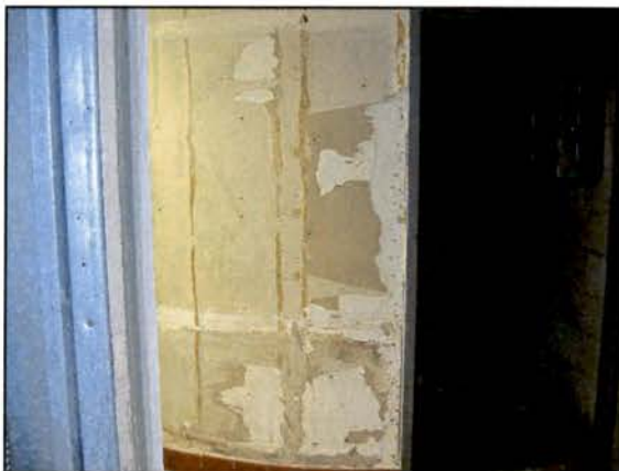
Gypsum Wall Board with Tape and Joint Compound, Newer and Gold Adhesive Residue (Samples 7A and 13A)
