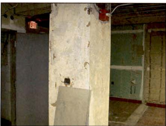
Column Plaster (Sample 3D)
