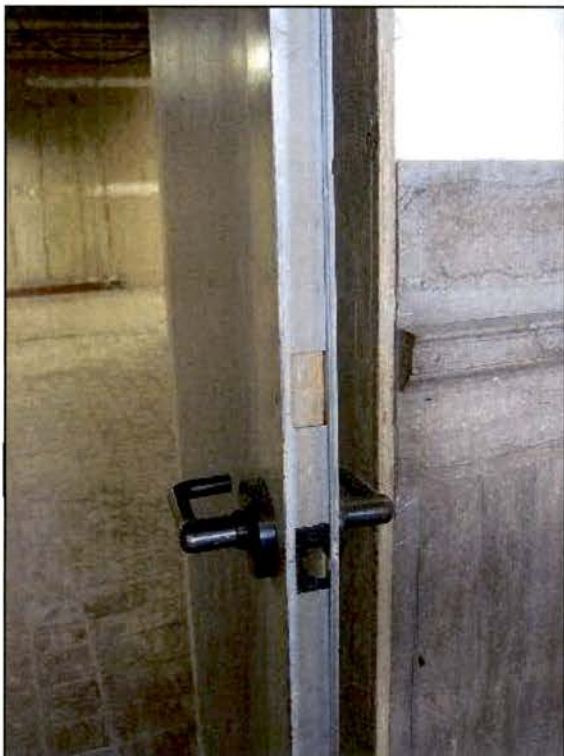
Wood Door Interior (No suspect asbestos containing materials)
