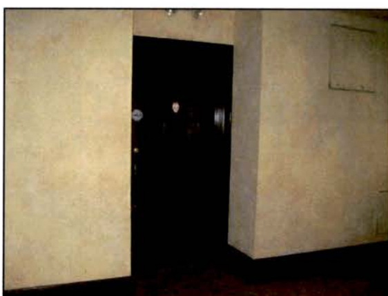
Mezzanine – Wall Texture (Samples 22A-C)
