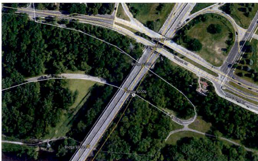
Figure 3 – Seventh Street AOI Bridges
