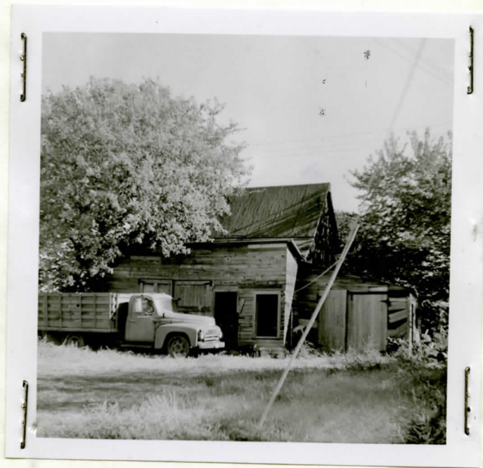
Garage & Storage Shed
