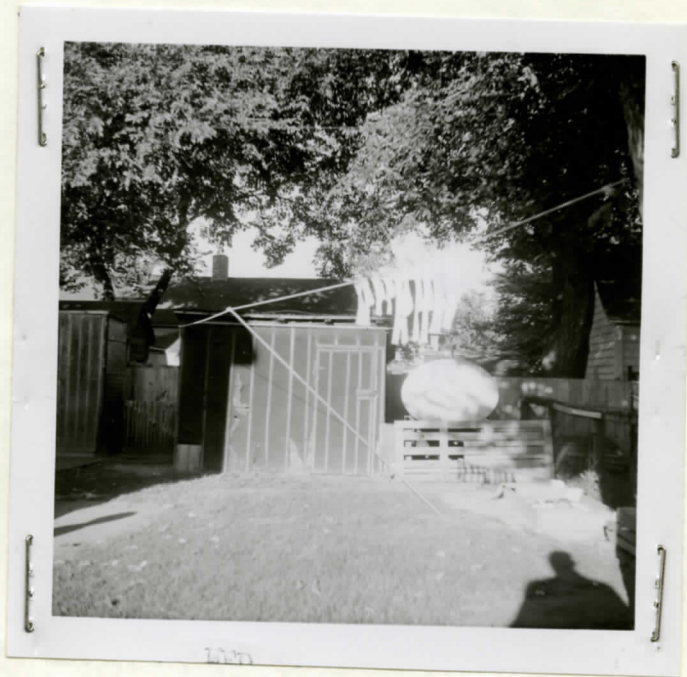
Shed on rear of lot
