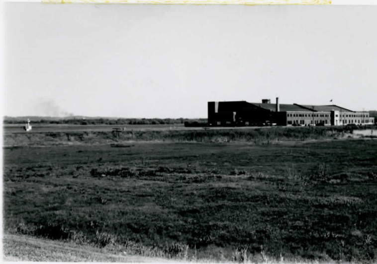
View of Subject Property from Airport Road looking southeasterly
