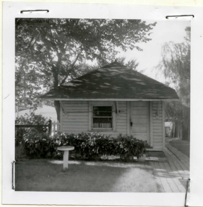
STORAGE SHED and GARAGE
