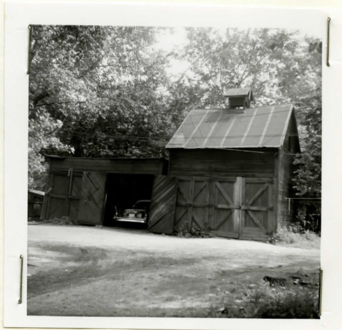
SHED AND GARAGE
