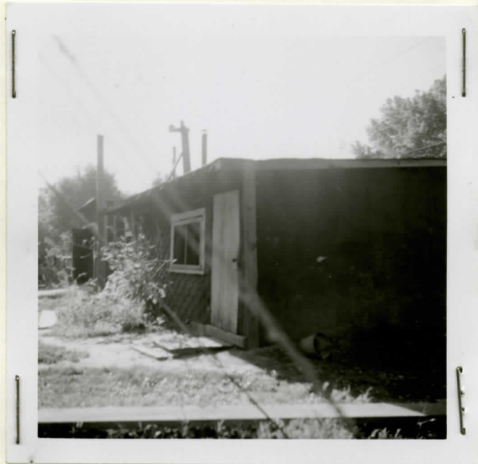
Shed on rear of lot
