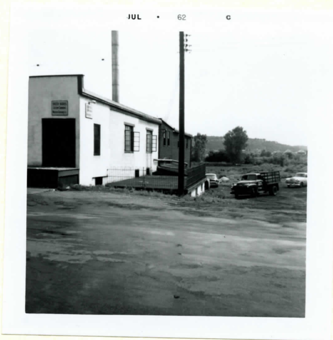
South Side of Building from the Front
