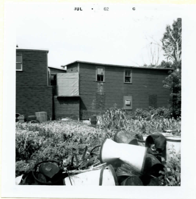
Rear Portion of Building
