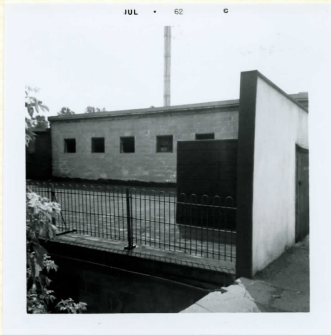
North Portion of Building
