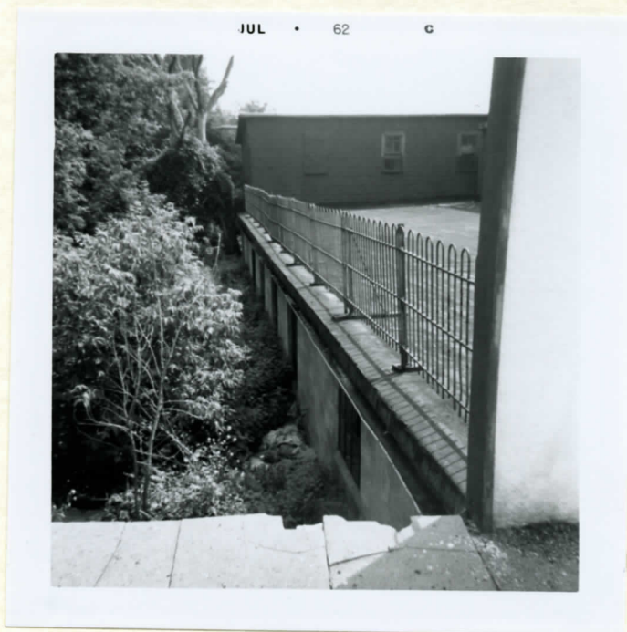
North Side and Showing Part of the Rear Portion of Building
