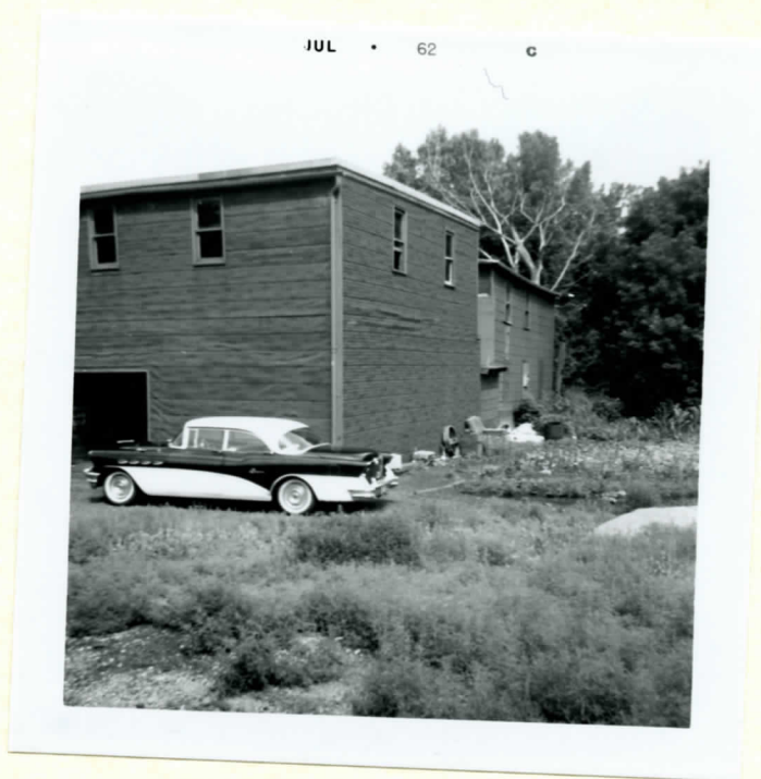
Rear Portion of Building
