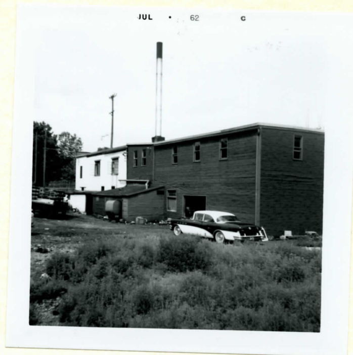
South Side of Building from the Rear
