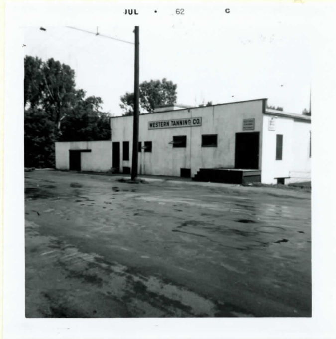
Front of Building - Facing State Street
