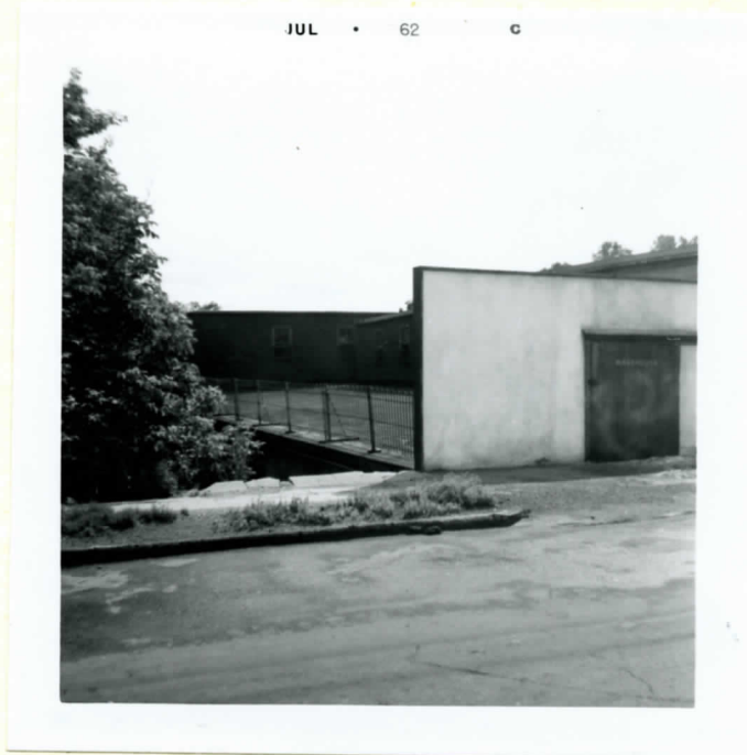
North and Front Portion of Building
